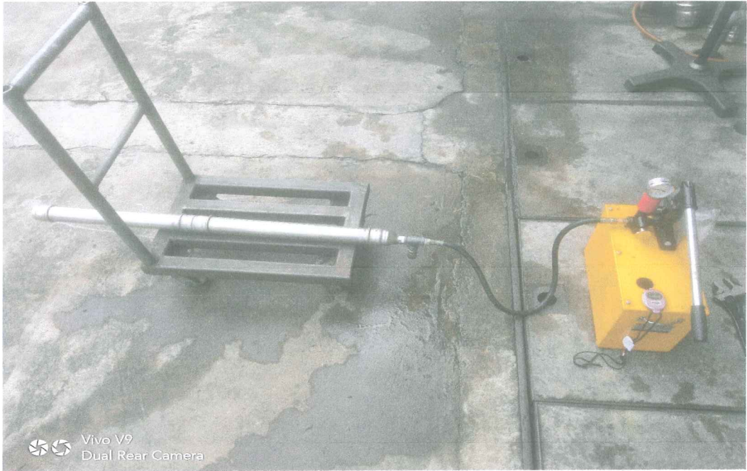
Hydrostatic Test Setup in Progress
